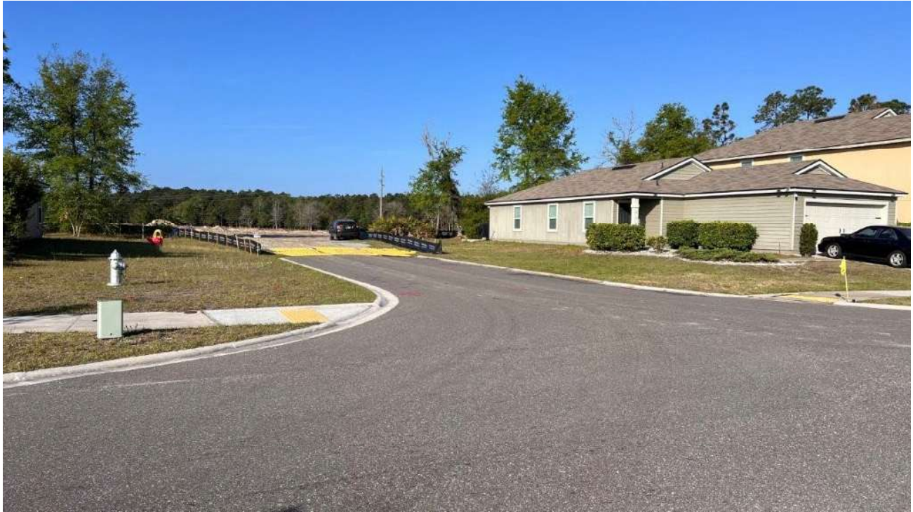
Missing stop sign and stop bar on Acorn Creek Road at the Intersection of Buck Creek Place
