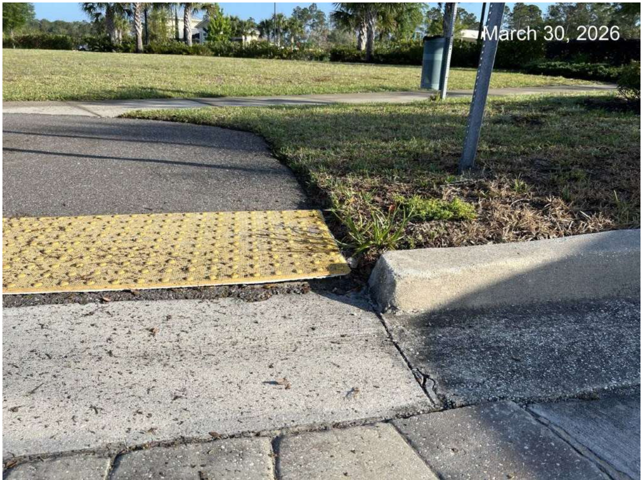
Raised ADA mat at Amenity Center crosswalk near roundabout
