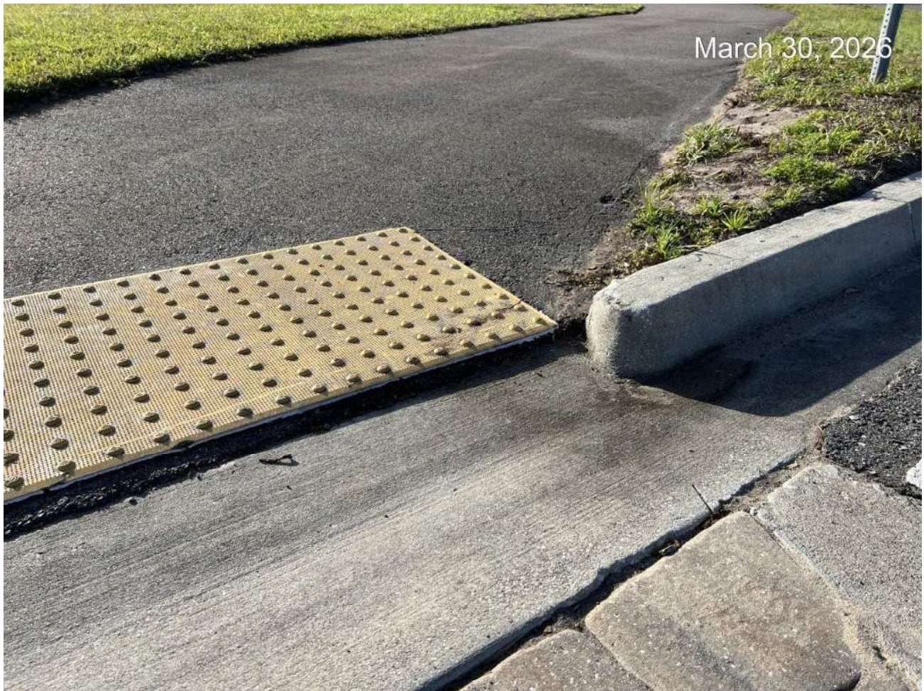
2 nd raised ADA mat at Amenity Center crosswalk near roundabout
