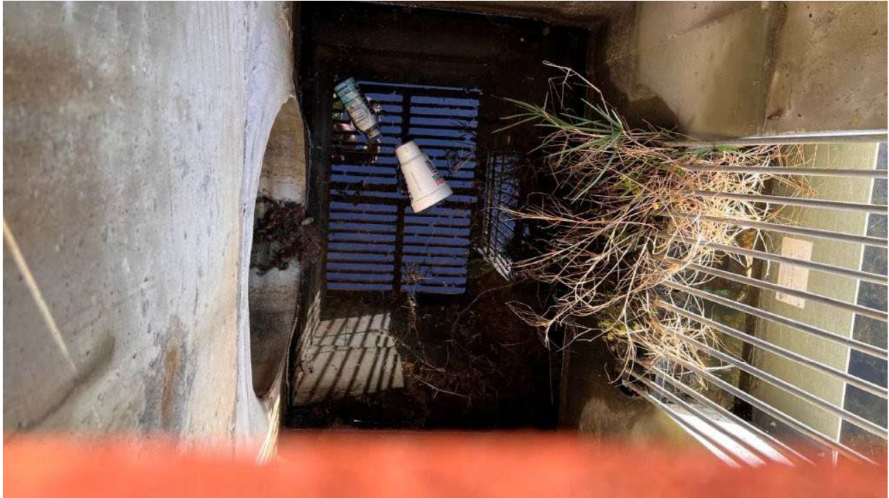
Control Structure for SMF 204 (Pond 6)
